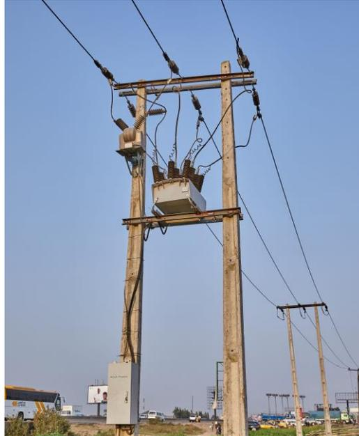
*Ikeja Electric NOJA Power OSM Recloser installation, using a H-Pole arrangement*
