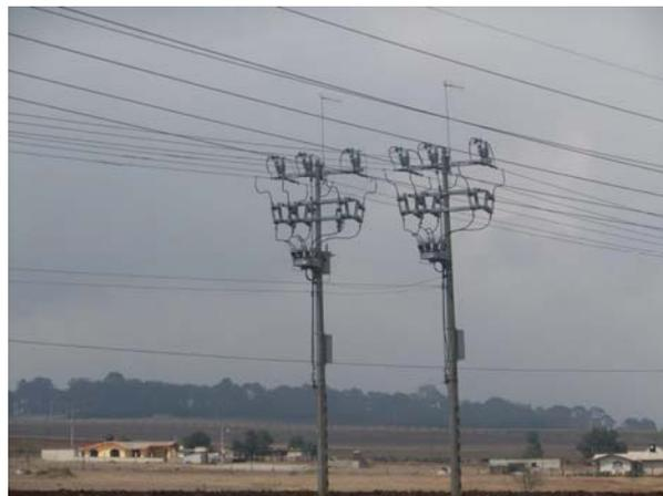
*Two NOJA Power OSM Recloser Installations on Parallel Feeders*
