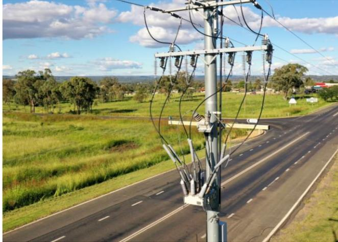
A [sectionaliser](#) is an automatic switch that opens when the power lines are not energized to isolate faulted sections .
